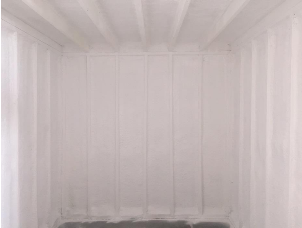
Figure 2. Example of application where DC 315 (white) serves as the thermal barrier over MD spray urethane cavity insulation (and overexposed studs/joists) 1 in wood-frame basement walls and ceiling.
